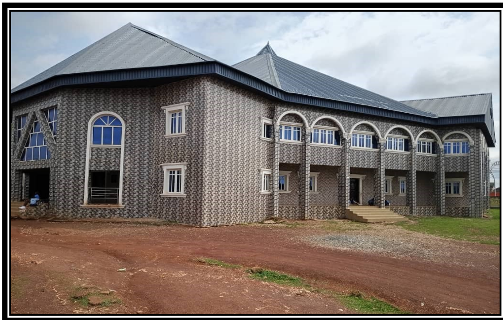
Figure 1: Showing the South-East view St. Andrew's Presbyterian Church, Azuiyokwu Model Parish, Abakaliki. (Source: Author's Field Work)
