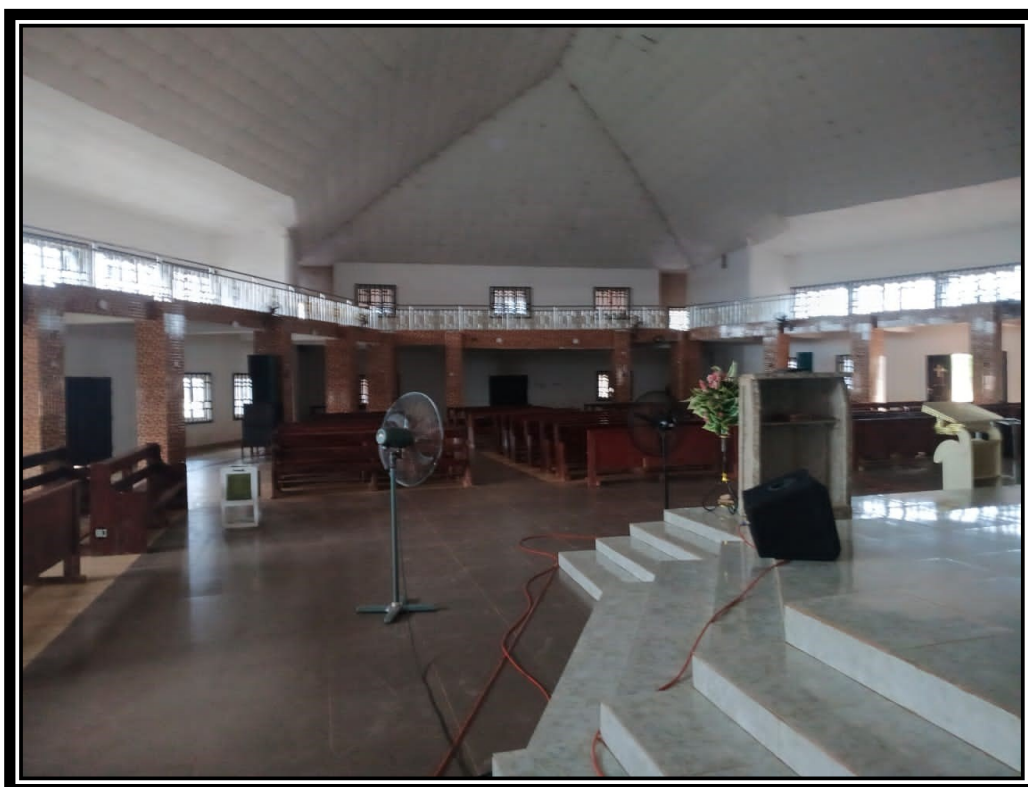
Figure 2: showing the interior perspective of St. Andrew's Presbyterian Church, Azuiyokwu Model Parish, Abakaliki, with floor finished with Tiles and plastered sandcrete block wall ( Source: Author's Field Work)
