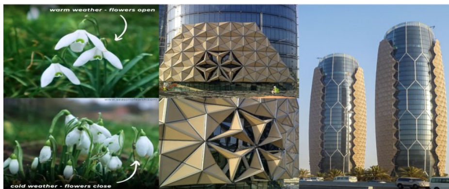
Figure 2. Snowdrop opened when warm and closed when cold (left), the mashrabiya-inspired facade (middle), and the Al Bahr Towers (right). Process Level Biomimicry. Source: Compiled by authors (2025).
